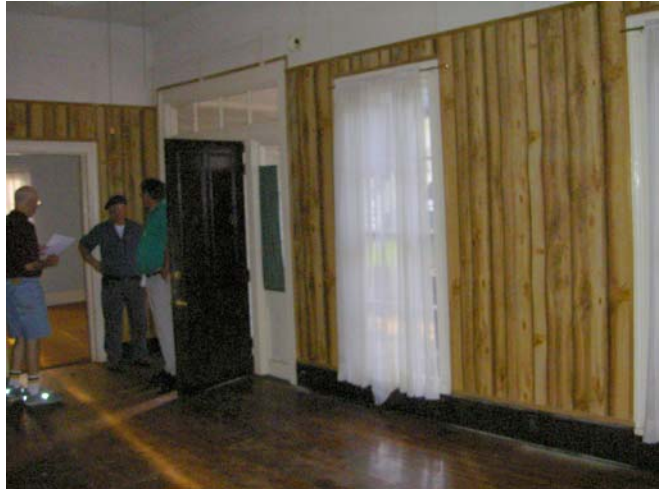
More Pictures of the Inside before the Interior Tear out Work Begins
